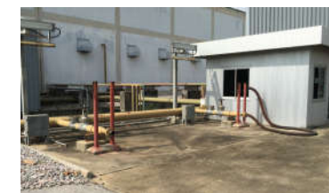
Diesel Unloading Station Thermal Power Plant
